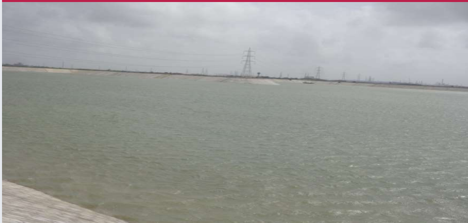
Raw Water Reservoir
